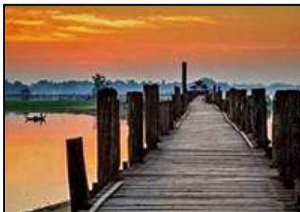
U Bein Bridge Myanmar
